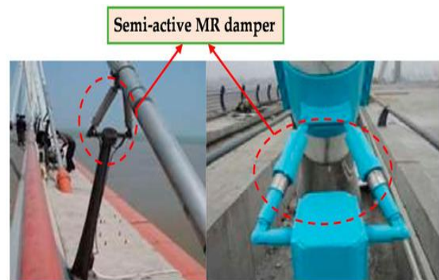
Fig. 6. MR Damper Application
